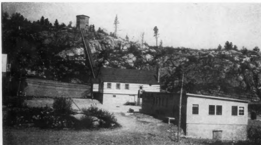
• • • Water tower, dining hall, office and warehouse buildings.
